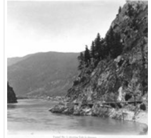
18. Tunnel No. 1, showing Yale in distance
