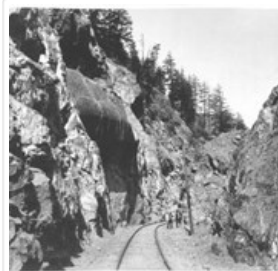
32. Rock cut between Tunnels 15 and 16, Cisco
