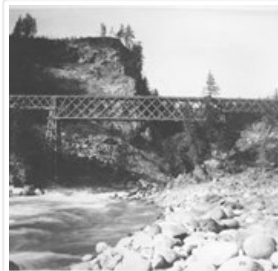
64. Salmon River Bridge, 200 ft. span
