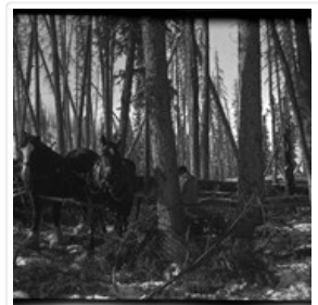
Elliott Barnes clearing timber on his Jumping Pound homestead
