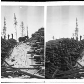
Men and team stacking timber
