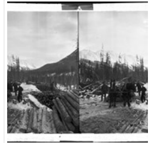
Men and team stacking timber
