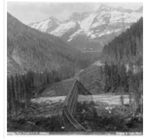
1017. The Loop showing four tracks, C.P.R. (Selkirks)
