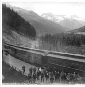
670. C.P.R. Express crossing Stoney Creek Bridge
