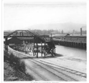
254. Foot Bridge & C.P.R. Station, Vancouver
