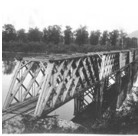
78. Harrison River Bridge
