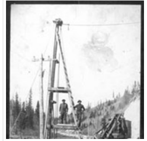
569. Pile driving on Columbia, B.C.
