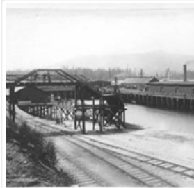
254. Foot Bridge & C.P.R. Station, Vancouver
