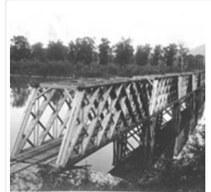
78. Harrison River Bridge
