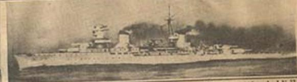
ITALY: The speedy new 6791-ton cruiser, "Giuseppe Garibaldi," with eight 6-inch guns in four turrets and a speed of 36.5 knots.
