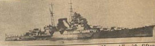
JAPAN: The new 8,500-ton cruiser, "Mogami," with fifteen 6-inch guns in five triple turrets and a speed of 33 knots.
