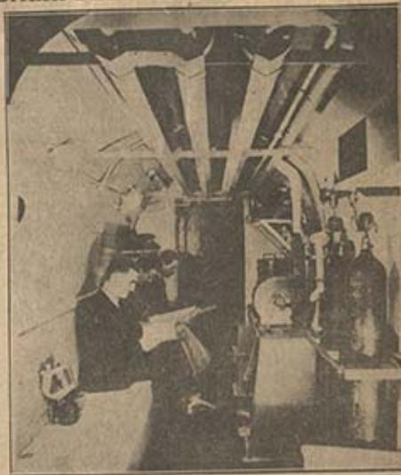
A view of the interior of a gas chamber recently installed by a London firm for the protection of its employees in the event of gas raids over the English metropolis. The chamber is proof against every known form of gas and is equipped with air filters, first-aid station, food lockers and water supply. The chamber has its system of communication with the outside world by radio and telephone.
