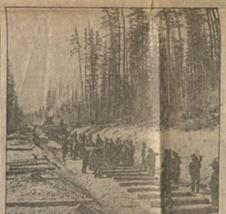
Tough work: Laborers carry cross ties from supply trains in the Lower Fraser Valley to the construction site. This grew started work on a B.C. section of the line in 1880.
