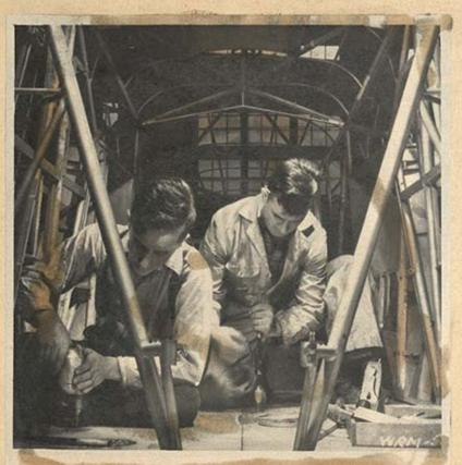
HERE IS A GLIMPSE inside a fuselage skeleton on the primary assembly line at Noorduyn, showing workmen applying flooring to the cabin area. Besides the training planes being turned out at Noorduyn, other Canadian factories are making fighter planes and long-range bombers for use in Britain
