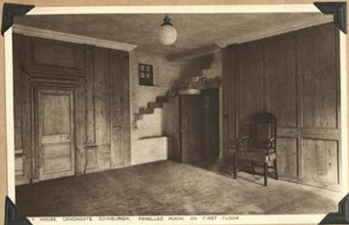
HOUSE, CANONGATE, EDINBURGH, PANELLED ROOM, ON FIRST FLOOR
